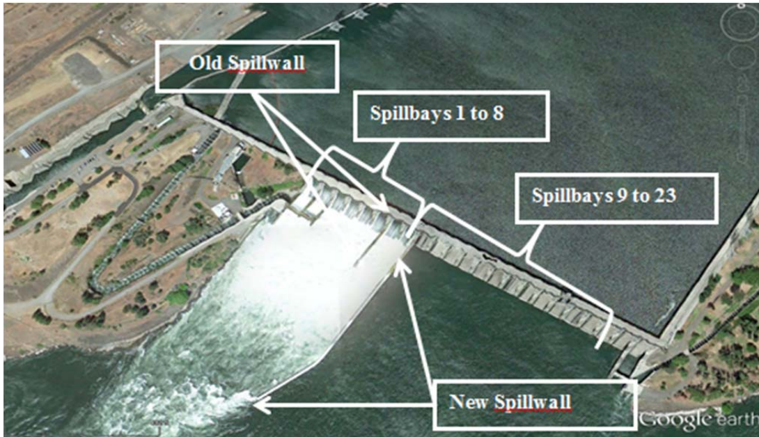
Figure 1.2. TDA Study Area Photo Showing TDA Spillbays and Spill Walls. A modified image (45°36'49.19"N, 121°8'0.61"W) from Google Earth™ (V7.1.2.2041), Google Inc. (Accessed October 14, 2013).
